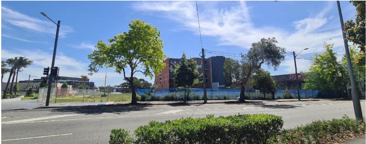
Figure 3: View looking west, of the subject site at the western frontage to Botany Road
